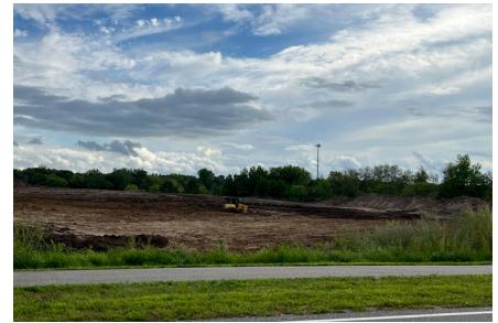
Earthwork progress in August
